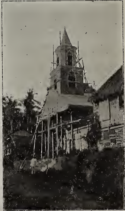
NEW CHAPEL AT PAGSANJAN IN PROCESS, OF CONSTRUCTION
